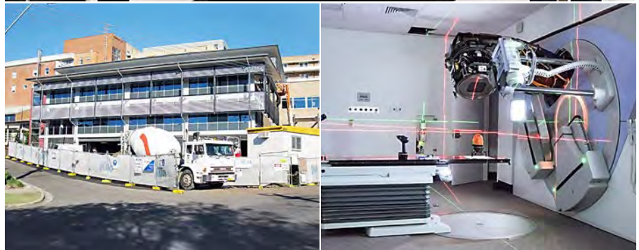
Top, from left, University of Newcastle student Daniel Lowe, NCCI Chief Radiation Therapist Stephen Manley, Radiation Therapist Patrick Magee and Radiation Oncologist Dr Shreya Armstrong with the new Surface Guided Radiation Therapy System. Bottom, construction of the NCCI, and installation of the LINAC in 2010
